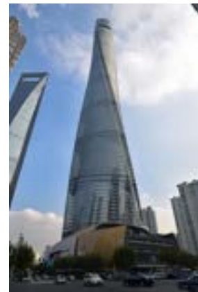
(F) Shanghai Tower, Shanghai.
