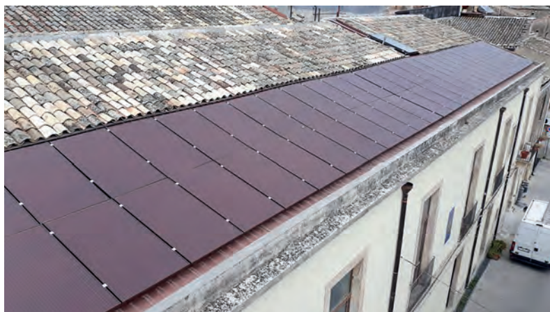
FIG. 9 View of the roof of the Ferla auditorium with the photovoltaic array with coloured, integrated panels (Municipality of Ferla).
