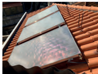
FIG. 7 Insertion of solar collectors during a renovation in the HCP. This type of action is allowed and recommended in the Guide, as not visible from the street, but the “granular” multiplication of such devices certainly will have greater impacts of scale on the Historic Urban Landscape.
