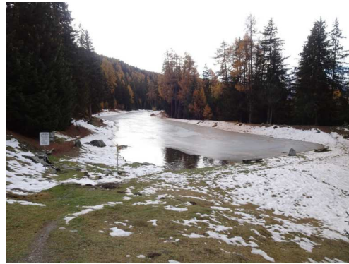
The Lac de Vernamiège, built by damming the small hollow between the moraine ridge (on the right) and the slope (ph. Andrea Ferrando)
