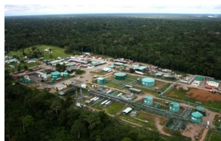
Figure 2. Sansahuari Pumping Station
