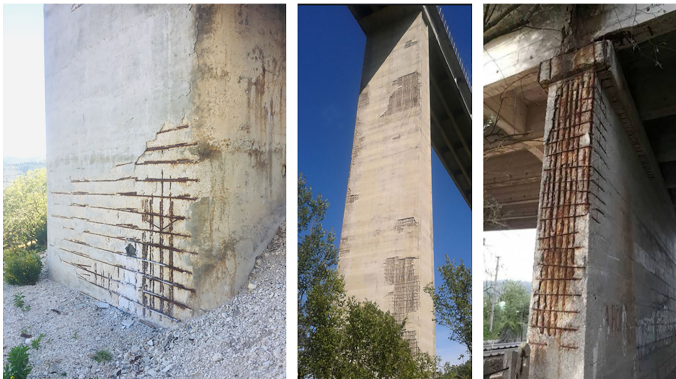
FIGURE 1 Examples of RC bridge piers subject to spatially non-uniform corrosion.
