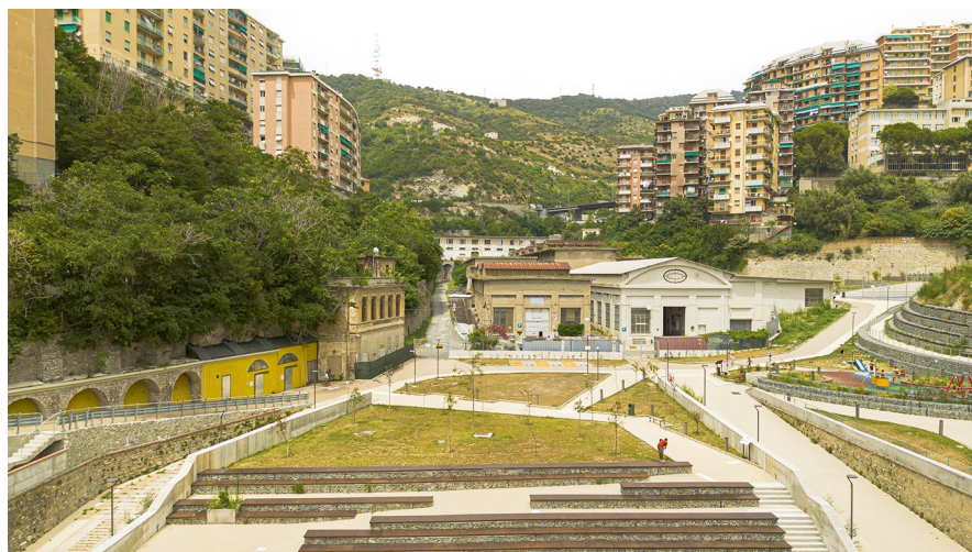
Fig. 7.7 Gavoglio Urban Park with 12 NbS in the city of Genoa (Italy, 2023), southern area activities are implemented to evaluate the performances in terms
