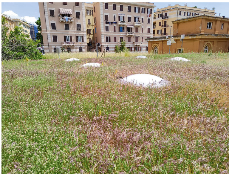
Fig. 7.3 Green Roof in Genoa (Italy) on DICCA, University of Genoa, with low management and high level of biodiversity
