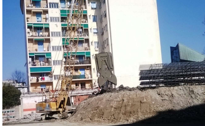
Figure 2.12 Diaphragm wall construction.
