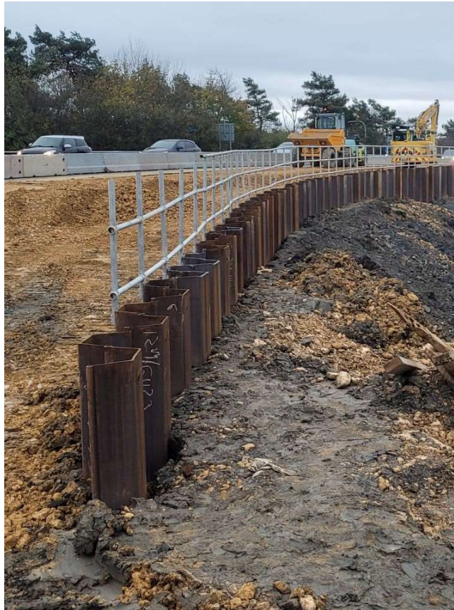
Figure 2.8 Example of steel sheet-pile wall
