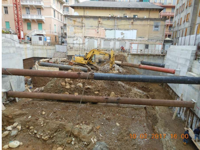
Figure 2.19 Example of excavation with struts
