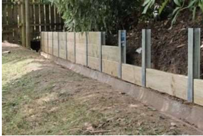
Figure 2.14 Example of King post wall
