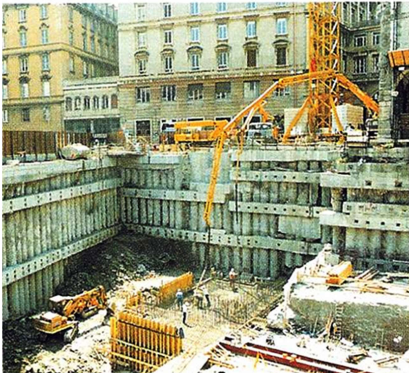
Figure 2.10 Example of excavation sustained by bored-pile walls
