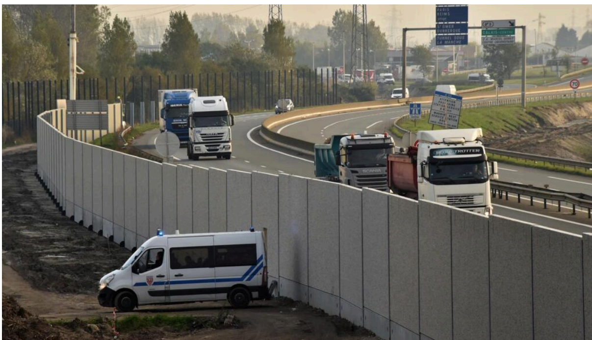
Fig 6. UK-funded walls and fences built around Calais region to block access to highways. © HRO
