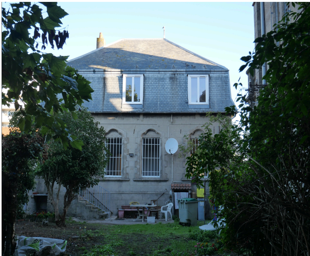
Fig 12. Emergency shelter in Calais. © Ismail Oubad
