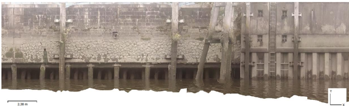
Figure 51. A sample of the 3D model of the quay wall. The screenshot was taken from Agisoft Metashape© (V 1.8.2).
