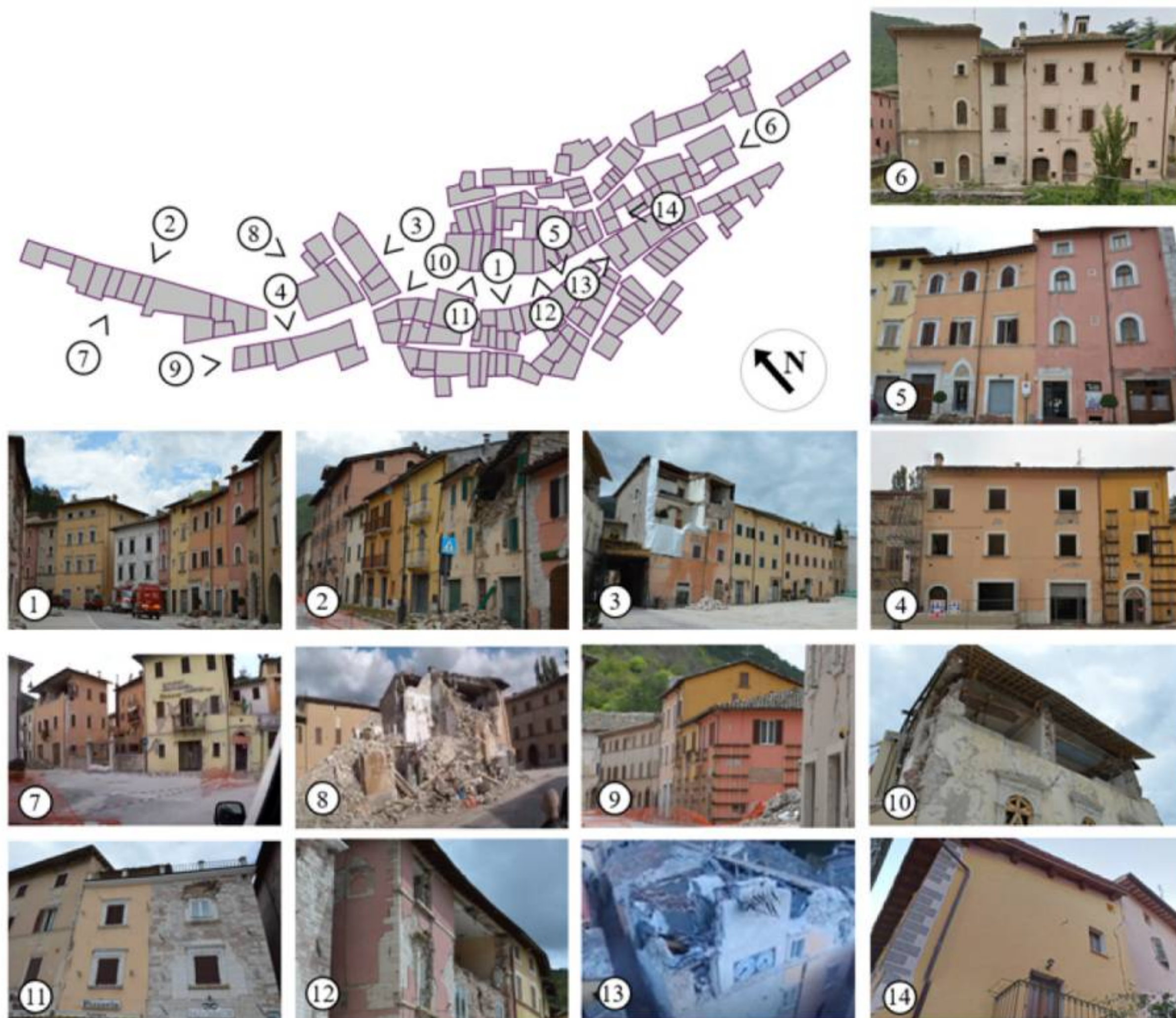
Fig. 11. Planimetric and photographic representation of the damage of the historic center of Visso.
