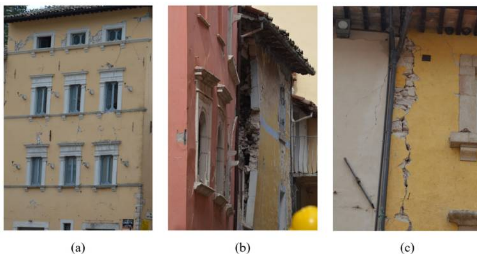
Fig. 3. Types of damage mechanisms: a) IP damage, b) OOP damage, c) damage from interaction between SUs.
