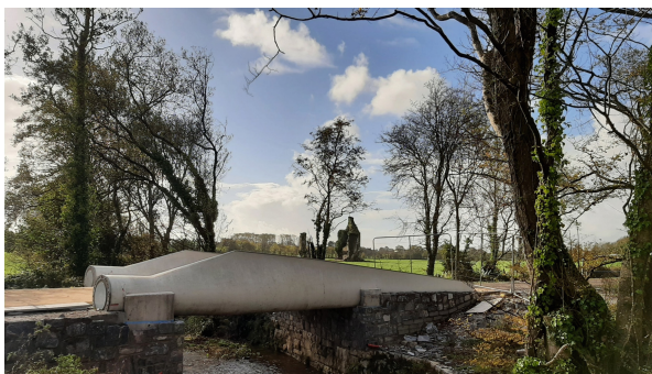
Fig. 1. Blade Bridge, Co.Cork, Ireland used for rapid assessment with Laser Doppler Vibrometry. The blade length is 11 m, the bridge span is 5 m and the maximum chord is ~1 m.
