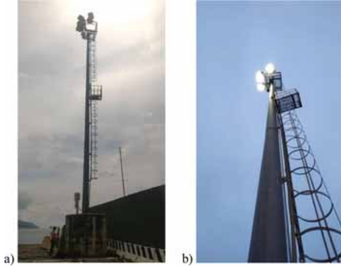
Fig. 1. Global view of the tower (a); the polygonal shafts composing the tower (b).
