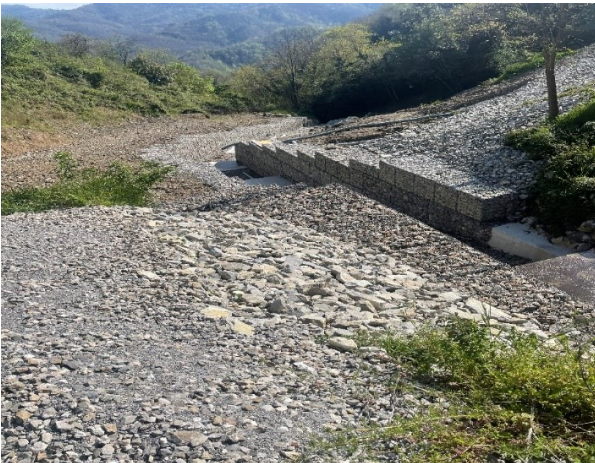
Figure 22: The gabion revetment system with six check weirs, lateral view (b)
