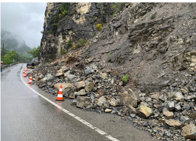
Figure 8: Rockfall along a municipal road in the Maritime Alps Department
