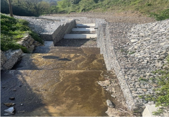
Figure 21: The gabion revetment system with six check weirs, front view (a)
