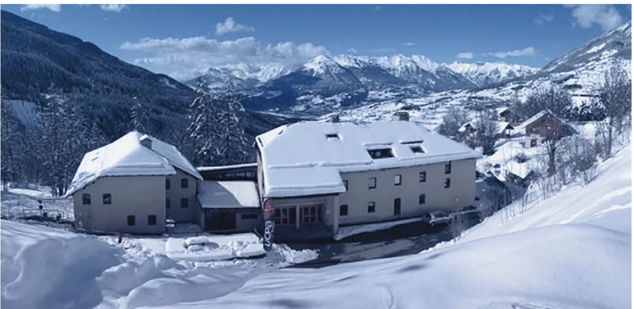
UCPA Center, newly equipped with an Intelligent Building Solution (Credit: © UCPA)
