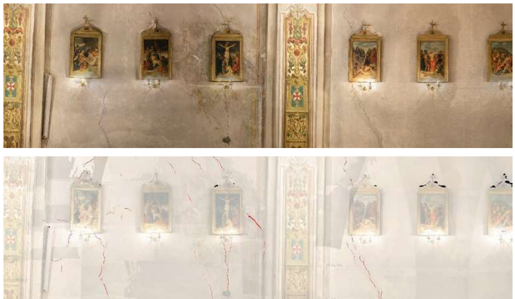
Fig. 8. SfM processing of the original images and their further processing in the Metashape environment using the algorithm.
