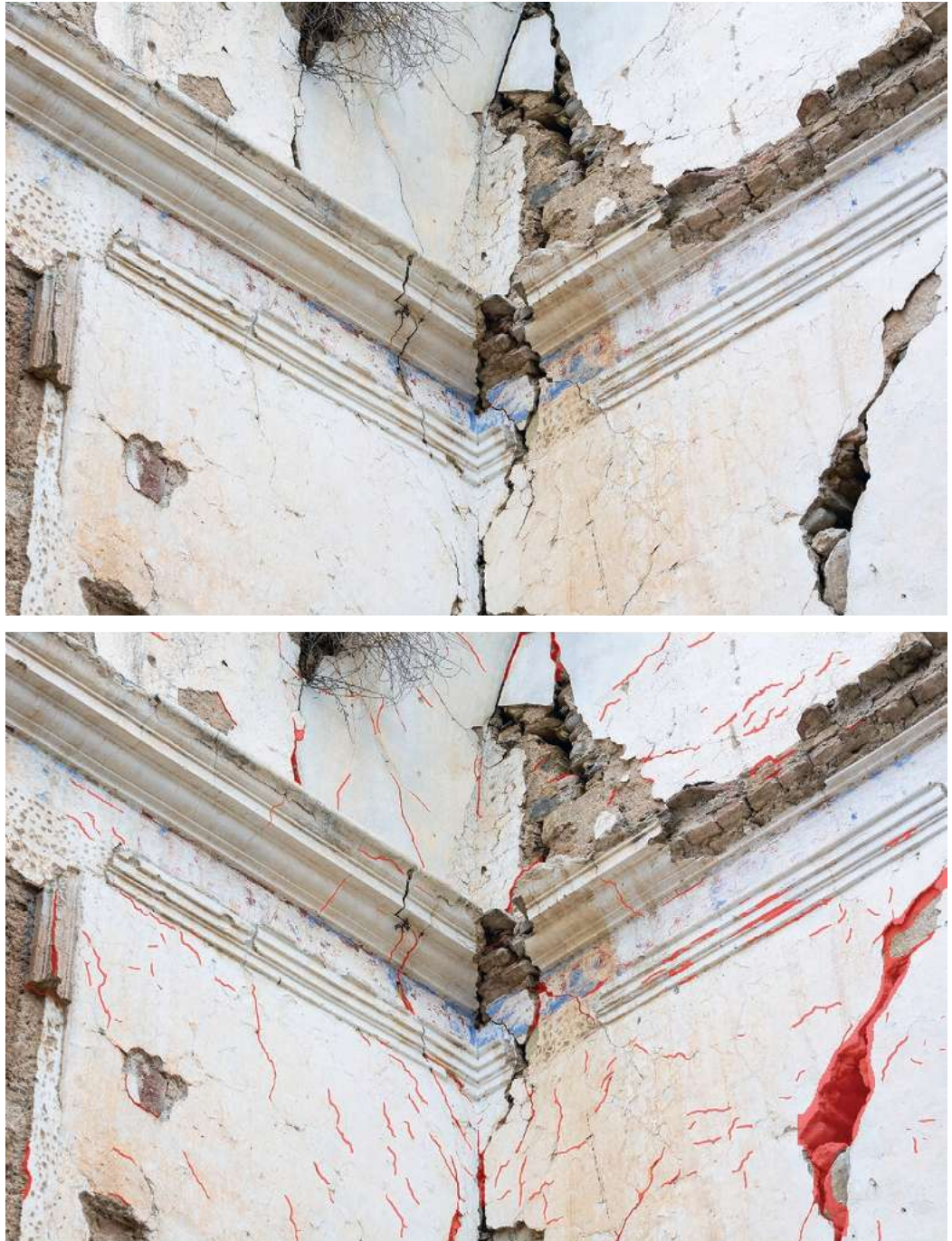
Fig. 4. On the left, the original image (photograph by the authors, 15 January 2023). On the right, the image processed using YOLOv11. Note how most of the cracks, shown in red, have been identified.
