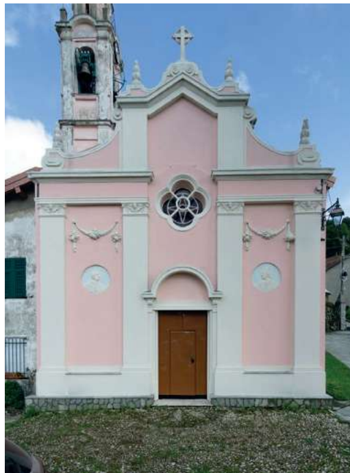
Fig. 7. On the left, a photograph of the main façade of the Church of San Carlo Borromeo in Cassingheno (photograph by G. Sacco, 3 October 2020). On the right, a schematic plan of the building.
