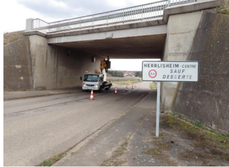
Fig. 1. Bridge monitored in both loadings and structural effects.
