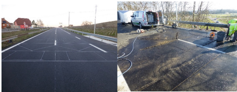
Fig. 2. Layout and installation of weigh-in-motion stations.
