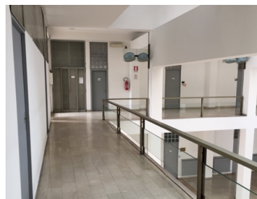
Fig. 3 – Gallery at the first floor (Photo by Sara Mauri, 2016)
