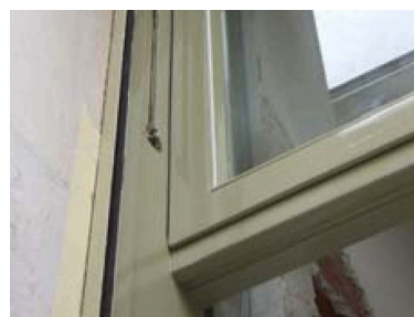
Fig. 9 – Detail of the restored sample window (Photo by Luca Ambrosini, 2006)
