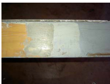
Fig. 7 – Stratigraphic analysis of the window wooden frame (Photo by Luca Ambrosini, 2005)
