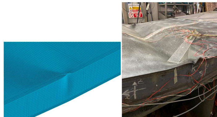
Fig. 28. Comparison between the numerical (a, left) and experimental (b, right) area of collapse.
