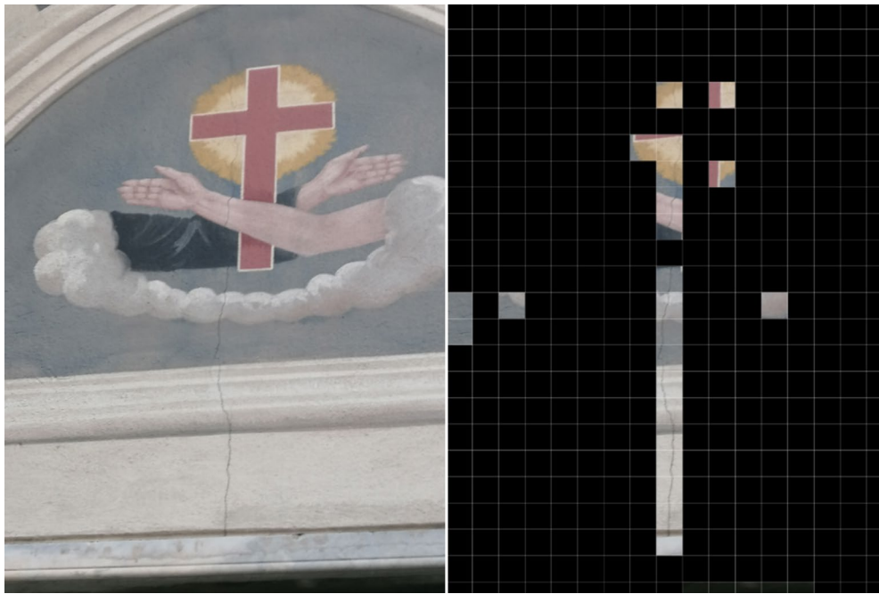
Fig. 19 Image of a decorated wall (on the left) and the corresponding image classified in crack patches and non-crack one, the latter represented in black (on the right)
