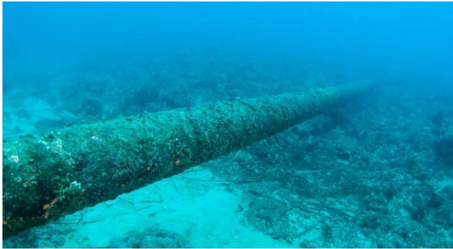
Figure 4.5 Pipeline Inspection Scene. Image credit: Satu Teknik Sdn Bhd.
