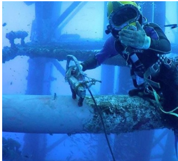
Figure 4.8 Manual Underwater Structure Inspection. Image credit: Aquatic Diving.
