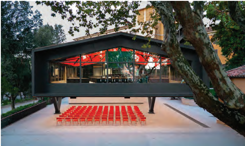
Figure 2 - The Dome. Designed by Alvisi Kirimoto in collaboration with Studio Gemma. Image ©Marco Cappelletti.
