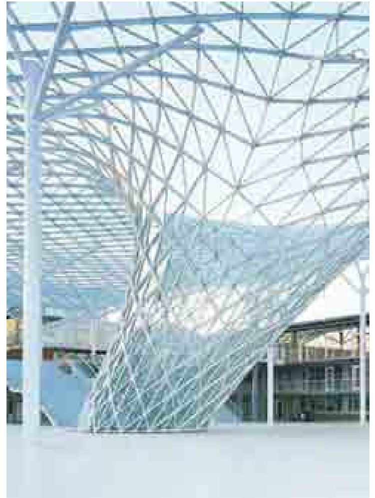
11.21. Precedent page: Actar Arquitectura: Communications tower, Turó de la Rovira (Barcelona, 2000). Above: Structural tornado for the New Milan Trade Fair. Massimiliano & Doriana Fuksas.
