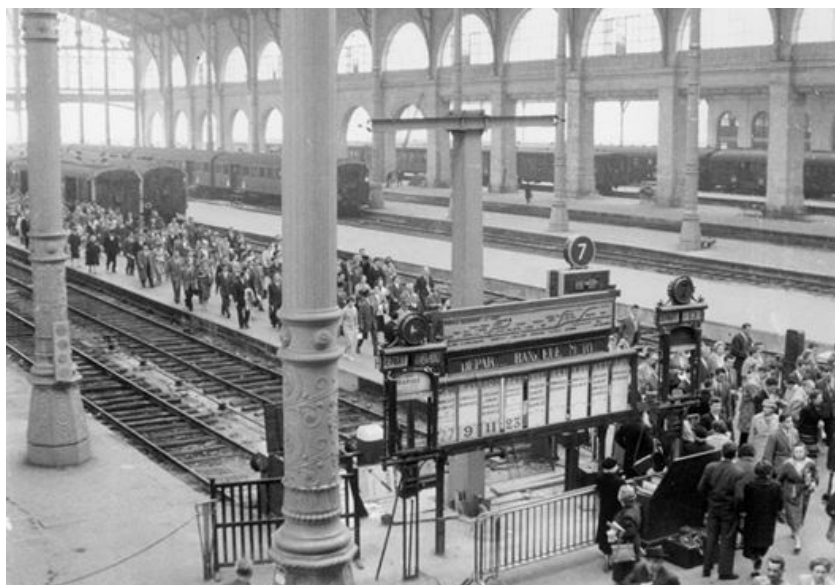
Figure 92 Picture of the creation of Gare du Nord II, approx. 1900
