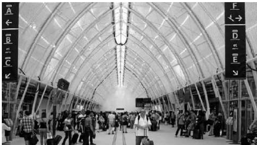
Figure 224 The new hallway at Montpellier Saint Roch
