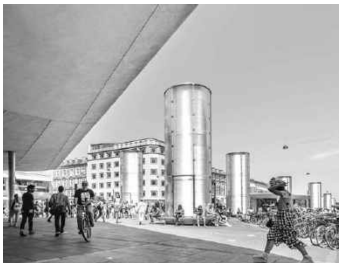
Figure 228 The ventilation pipes at Norreport Station
