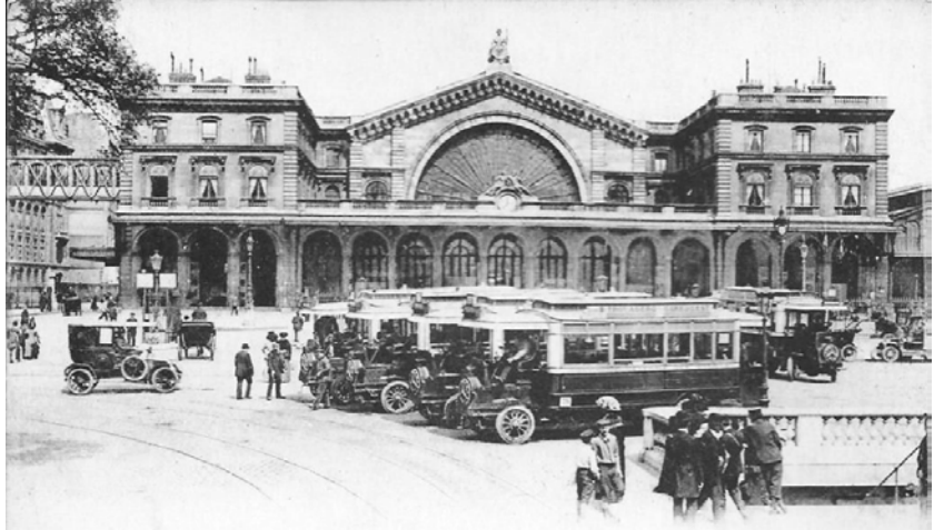
Figure 6 Old postcard showing the facade of Gare de l'Est from the metro entrance
