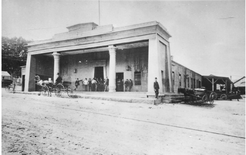
Figure 17 New Bedford station - 1886
