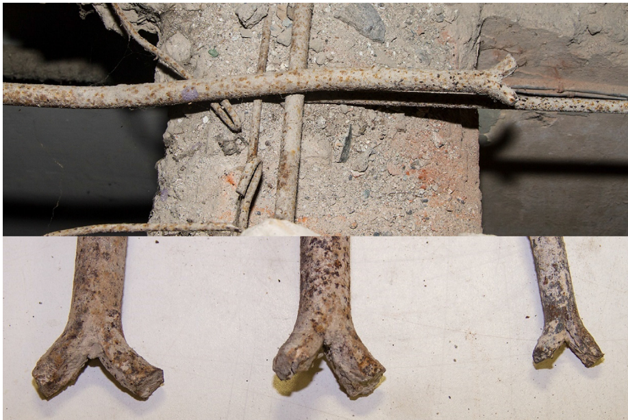
Fig. 2. Fish-tail ends and hooks of reinforcing bar of the slab of a villa inside the Villa Gruber park, Genoa (Italy), unknown building date, in-between 1900 and 1930.
