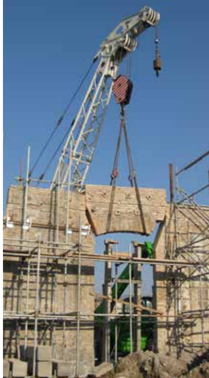
Prelievo dei singoli conci murari e degli architravi Removal of the blocks and of the architraves
