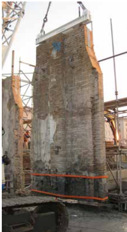
Prelievo dei singoli conci murari e degli architravi Removal of the blocks and of the architraves
