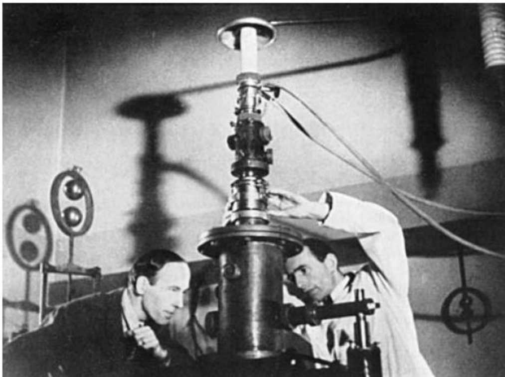
Figure 6.1 | The electron microscope built by Ruska (in the lab coat) and Knoll, in Berlin in the early 1930s. (Image from 184 )
