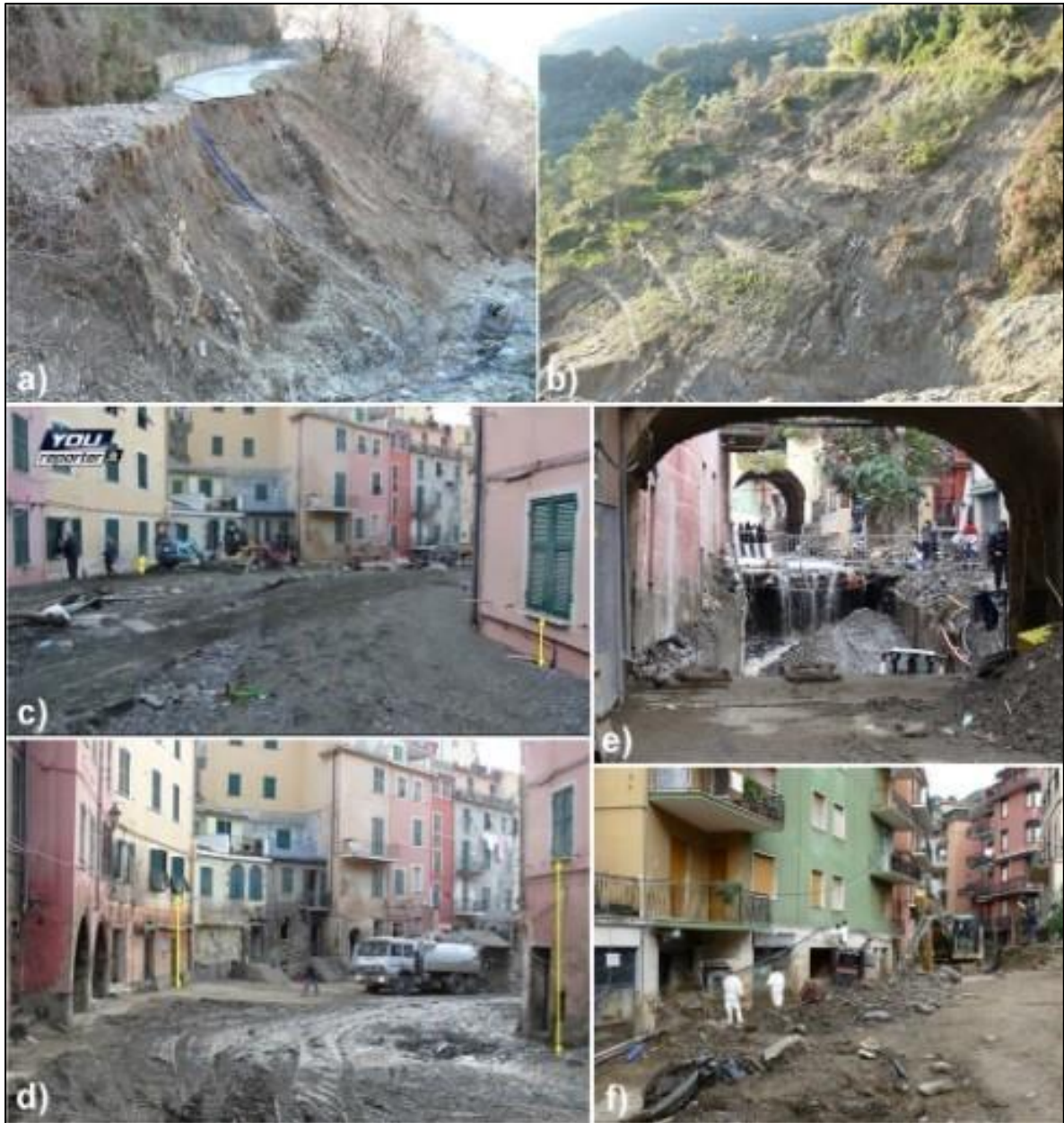
Figure 4.5 Some damage suffered in the Vernazza and Monterosso catchments due to the October 25 th 2011 precipitation (from Cevasco et al. 2015). a) Destruction of roads ( Vernazza basin); b) accelerated erosion on cultivated terraces ( Vernazza basin); c-d) the main street of Vernazza buried by mud and debris immediately after the rainfall (photo from http://www.youreporter.it , integrated) and after the removal of the debris flood deposits; e) destruction of a part of the covered tract of the Canale Pastanelli at Monterosso ; f) the main street of Monterosso during the works for removing the debris flood deposits.
