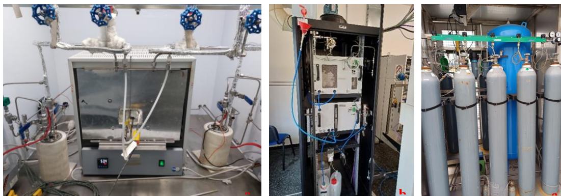
Figure 4-1 These are the main components of cell station 1. a) This section represents the central part of the setup. The furnace is located at the centre and houses the cell, which is inserted together with its cell frame. Gas lines from the flowmeters are connected to the cell from both the left and right sides. The two cylinders on both sides are the humidifiers. b) An AEM electrolyser, which provides hydrogen to cell station 1. c) The cylinders on the roof were initially both responsible for \text{CO}_2 and \text{N}_2 gases, successively only the \text{CO}_2 tanks were kept.
