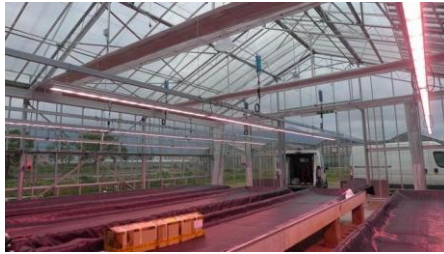
Figure 4.8 – LED lighting in the experimental greenhouse
