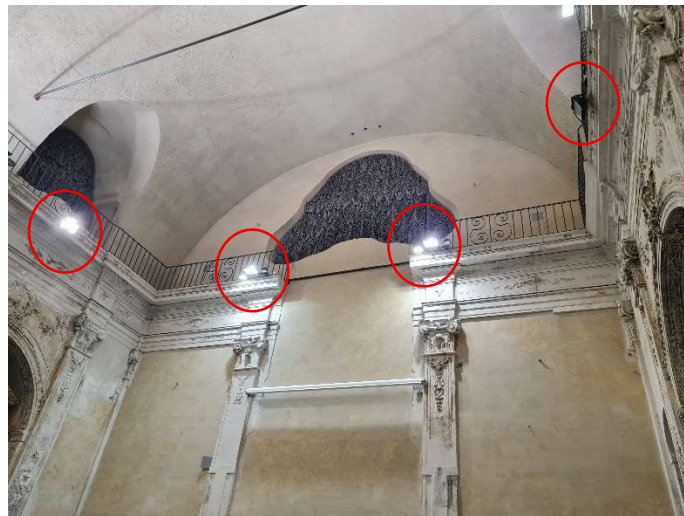
Figure 7. Lamps perceived as glaring or annoying by the students (red circles). The picture is a zoom of the lights over the speakers' stage visible in Figure 2.
